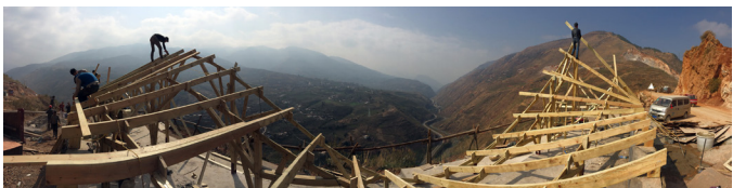
Figure 8: The Warp under construction
