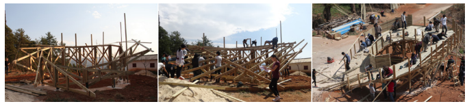
Figure 6: fabrication of trusses, ruled beams and ruled deck
