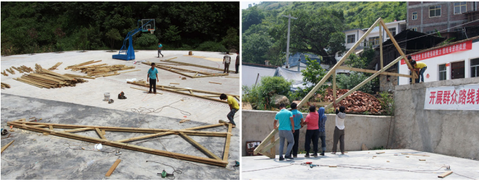
Figure 4: Prefabrication and installation of trusses on site
